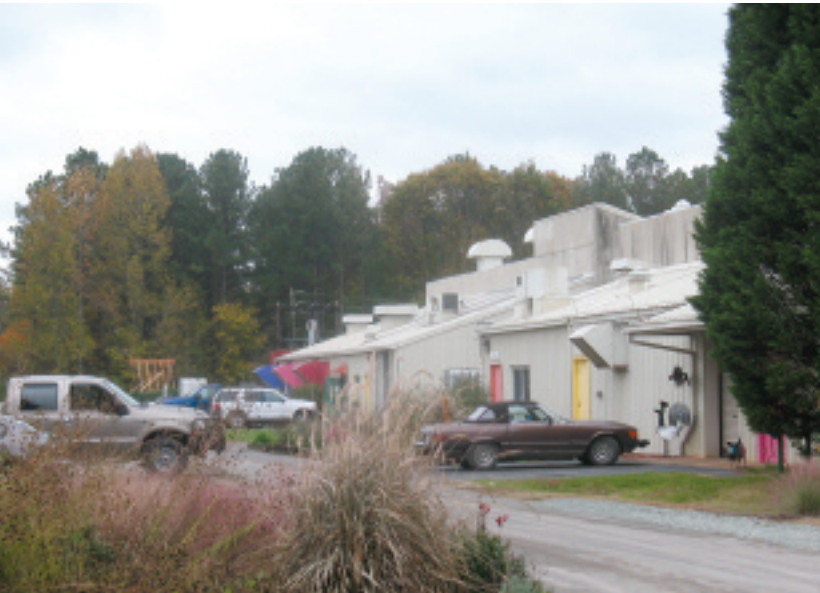
Piedmont Biofuels' commercial biodiesel processing facility in Pittsboro.
